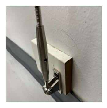
Bottom connection of cable guided system. Trim and crimp cable as required.
